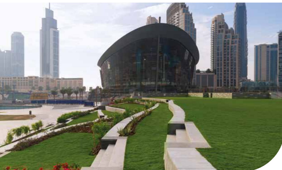
Dubai Opera (Utility house) - Burj Khalifa Complex, UAE
