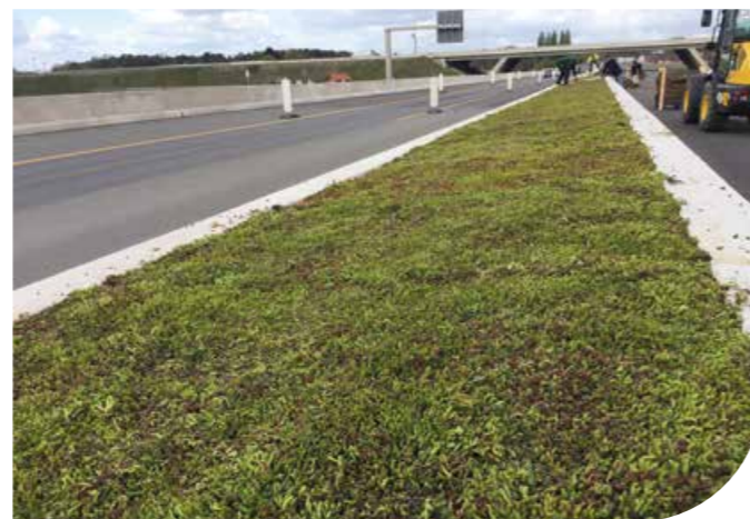
Highway belt on A33 motorway, Bielefeld, Germany
